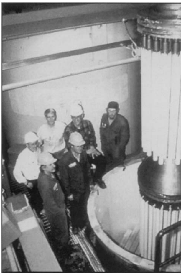
Figure 12-10. Westinghouse candle filter system, showing the hanging porous ceramic tubes. (Photo courtesy of Siemens Westinghouse, Pittsburgh, PA.)
